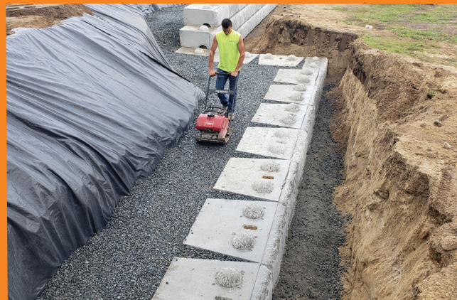
BROADALBIN TS RETAINING WALL
