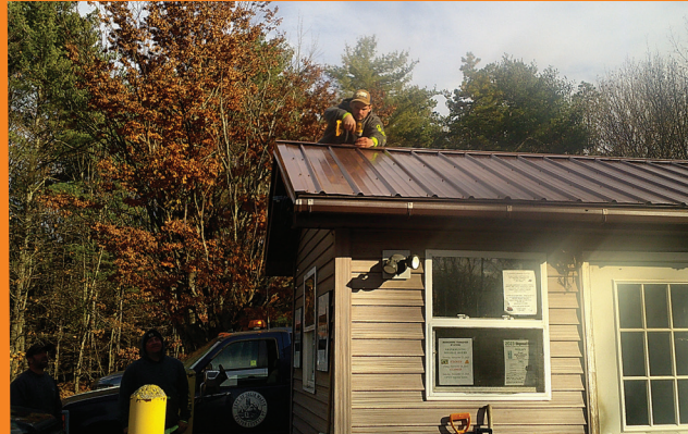
ROOF REPAIR AT BERKSHIRE TS
