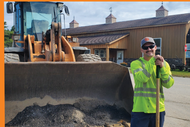
ROAD REPAIR AT DSW
