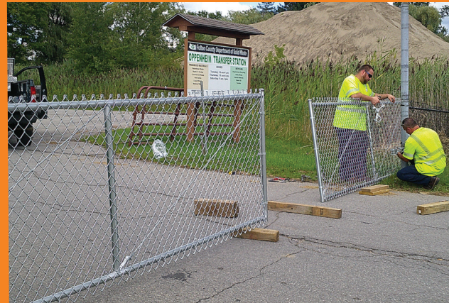
GATE INSTALL AT OPPENHEIM TS
